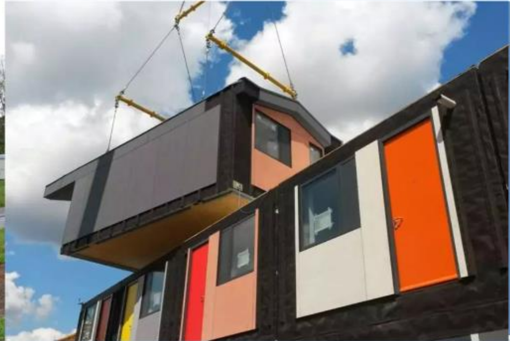
Fig 3: Assembling of modules in modular construction ( www.frozen.com )
