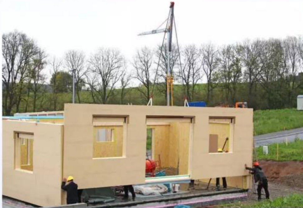
Fig 2: Assembling of panels in prefabricated construction ( www.frozen.com )
