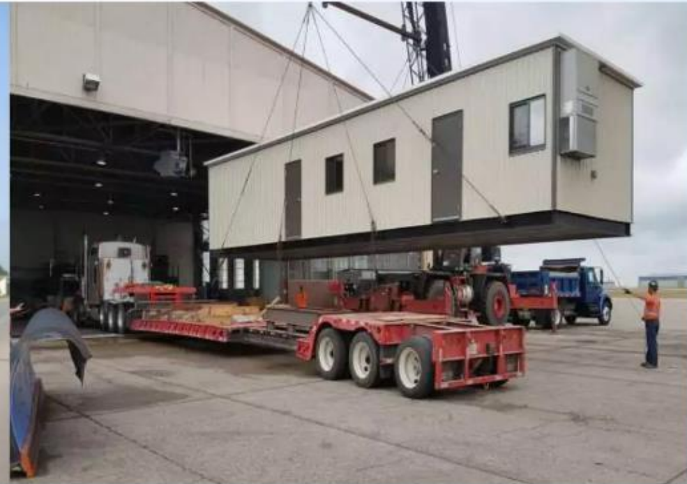
Fig 6: Placing building modules in trucks from the factory (Source:www.bennettig.in)
